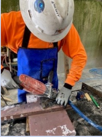
Adam Krapf drilling anchor holes.
